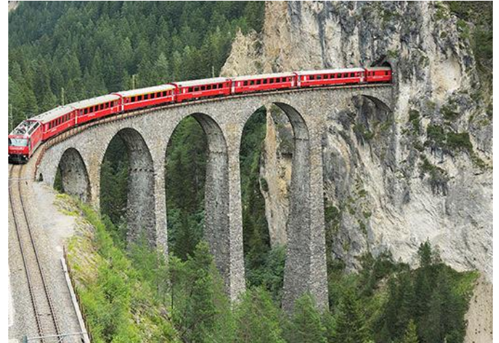
Railway viaduct in Switzerland, http://crea.bunshun.jp/articles/-/6770
