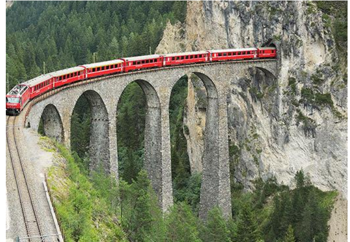
Railway viaduct in Switzerland, http://crea.bunshun.jp/articles/-/6770
