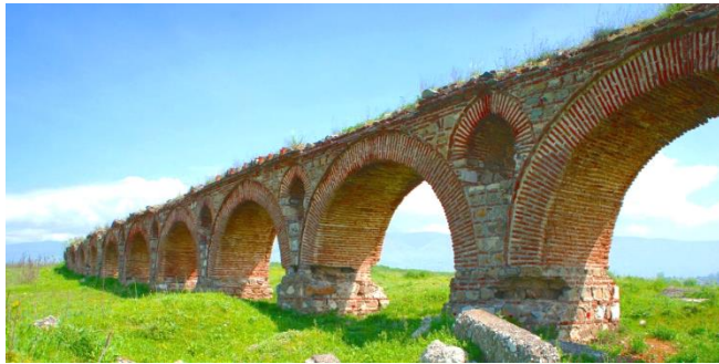
Skopje Aqueduct, Macedonia, 1st century; exploringmacedonia.com
