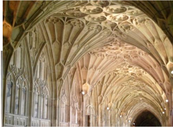
Gloucester Cathedral cloister walk, slideshare.net/michaelasanda/gloucester-cathedral2
