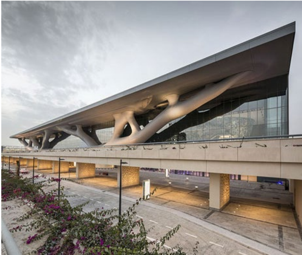
Gigantic tree-like columns support the overhanging roof canopy of the Qatar National Convention Centre by Japanese Architect Arata Isozaki
