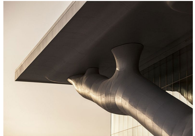
Gigantic tree-like columns support the overhanging roof canopy of the Qatar National Convention Centre by Japanese Architect Arata Isozaki
