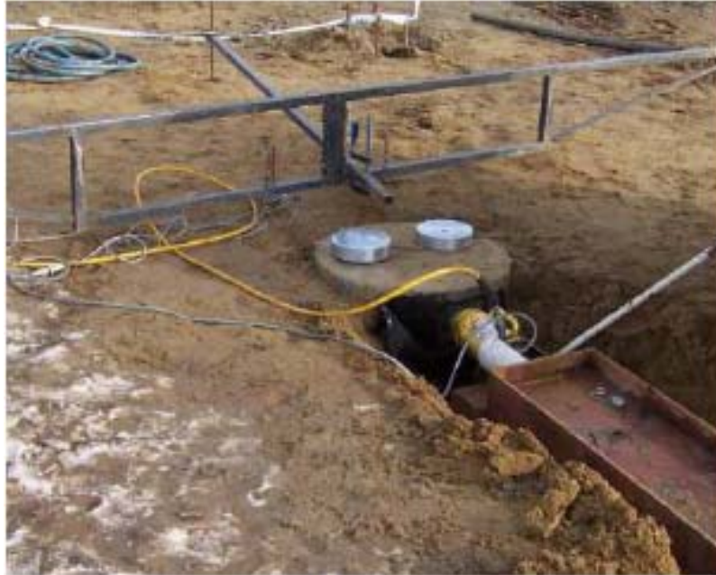
The test pile
